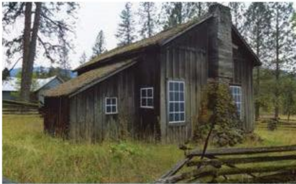
This building, built in 1861, was the McBeth missionary school. The US Forest Service in 1991 gave a new roof to the US Indian agent.
